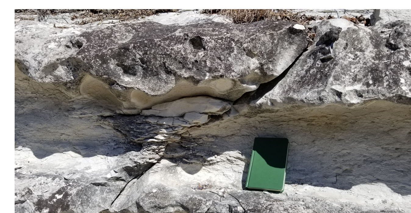
Figure 9. An example of a through-going fracture.
